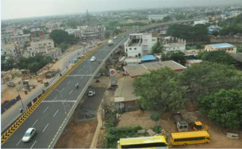
Grade Separator at Rettai Eri Junction on Chennai Inner Ring Road (Inaugurated by Hon'ble Chief Minister on 04.03.2017)
