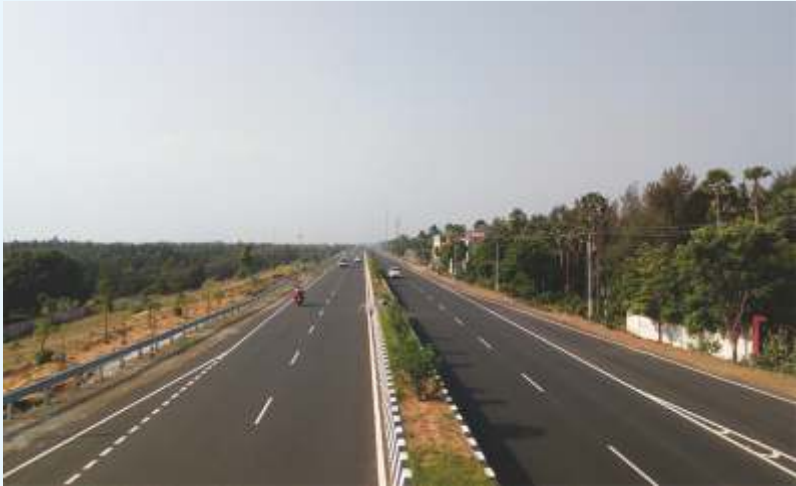
Four lanned East Coast Road from Akkarai to Mamallapuram
