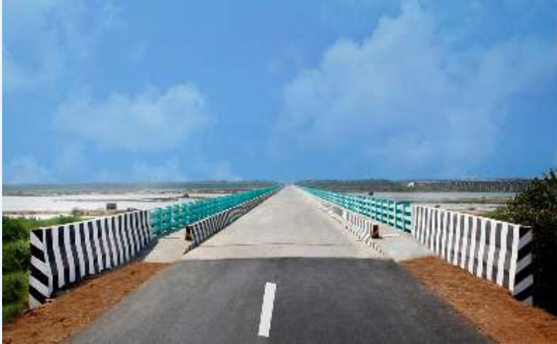
Bridge across Cauvery connecting Mohanur (Namakkal) and Vangal (Karur) inaugurated by the Hon'ble Chief Minister on 14.02.2016 (Longest River Bridge in TN)
