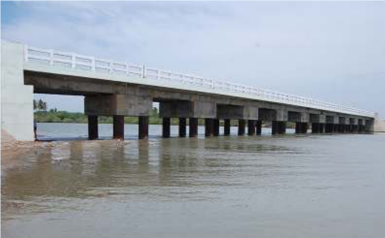
Edamanal-Thirunagari Bridge in Nagapattinam District (Inaugurated by Hon'ble Chief Minister on 07.03.2017)
