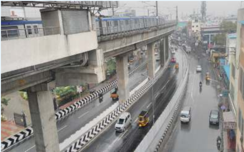
Grade Separator at Vadapalani Junction on Chennai Inner Ring Road (Inaugurated by Hon'ble Chief Minister on 04.03.2017)
