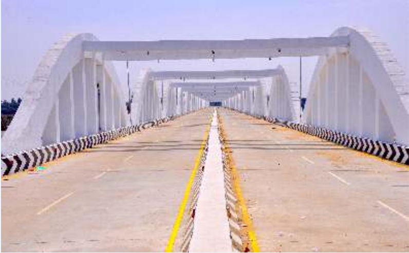
Bridge across Kollidam River at Srirangam in Trichy District (Inaugurated by the Hon'ble Chief Minister on 14.02.2016)
