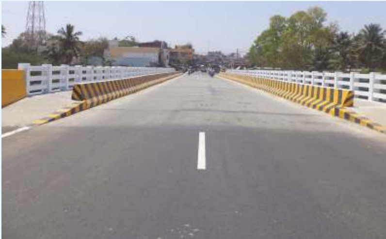
Bridge at Kambainallur in Dharmapuri District (Inaugurated by Hon'ble Chief Minister on 08.05.2017)
