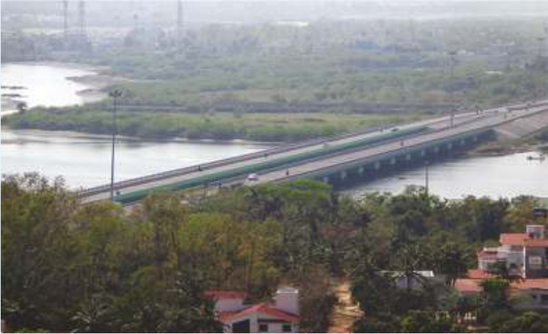
Additional Bridge at Muttukadu on East Coast Road
