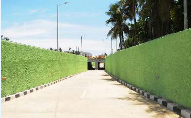
Limited Use Subway at Tiruvanaikaval in Trichy District (Inaugurated by Hon'ble Chief Minister on 07.03.2017)
