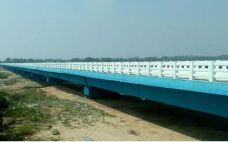
Bridge at Orakkattupettai in Kancheepuram District (Inaugurated by Hon'ble Chief Minister on 04.03.2017)
