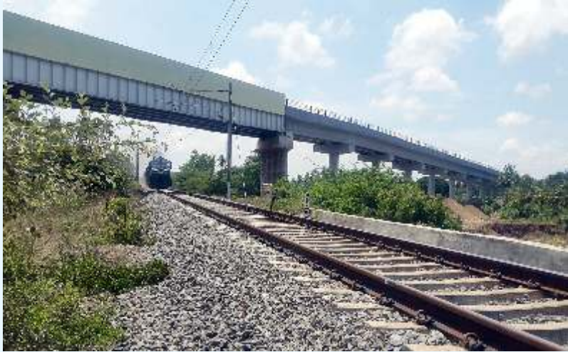
Railway Over Bridge at Singanallur in Coimbatore District (Inaugurated by Hon'ble Chief Minister on 18.03.2017)
