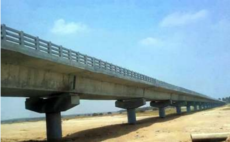
Bridge across Palar River connecting Thengal and Melvisharam in Vellore District
