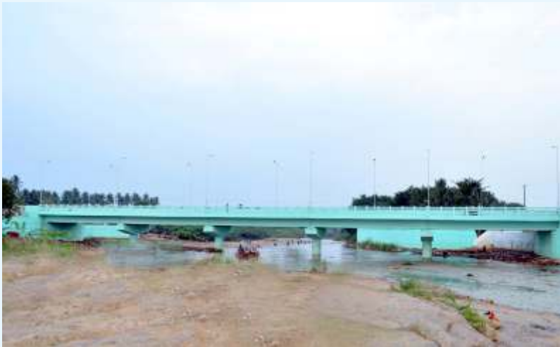
Amachiyapuram Bridge in Theni District (Inaugurated by Hon'ble Chief Minister on 14.02.2016)
