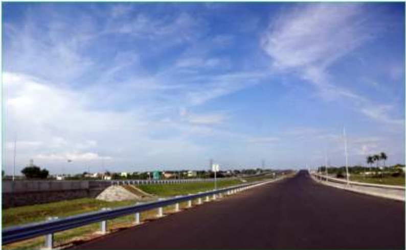
Chennai Outer Ring Road at Thennambakkam
